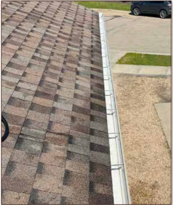
Cleaning out eavestroughs is one of the fall maintenance jobs that can help prepare a home for the winter months. Removing leaves and debris allows water to drain properly and helps prevent potential problems when snow and ice arrive.
