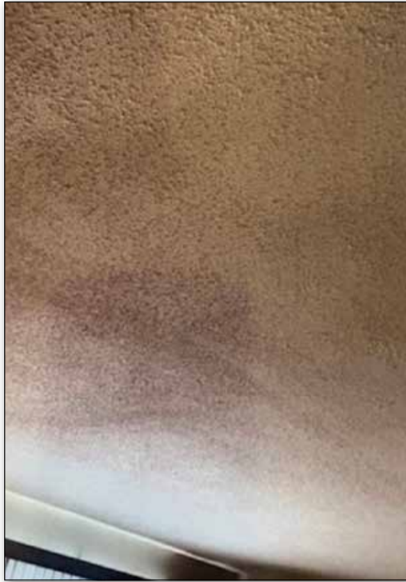
Sagging drywall in the living room ceiling is among the damage Sturgeon County resident Peter Pedgerachny says was caused by a series of earthquakes felt throughout the region earlier this spring.
