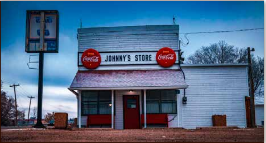
Built in 1902 and in the McNeilly family for generations, the iconic and historic Johnny's Store in Namao reopened with a new concept on Thursday, November 28, after four years of renovations and modernization. - Stephen Dafoe Photo
