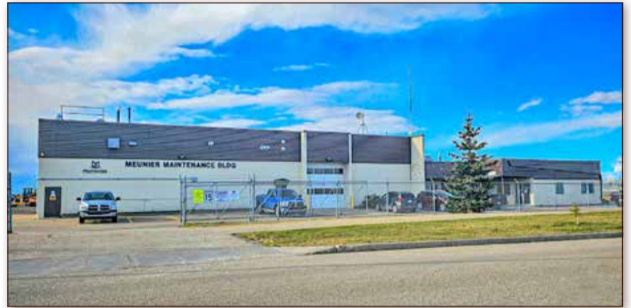
Morinville's Infrastructure Services Building, slated for potential $564,000 in repairs, awaits Council's final budget decision as discussions push funding and timelines further into future years.
